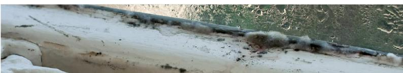
**Penetrating damp**. Rain may also seep through cracks in brickwork or through missing tiles on external roof surfaces, this would involve the brick work being re pointed and is rare within Leicester.
