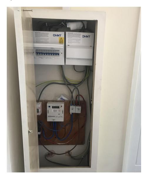
These circuit breakers are designed to cut out rather than 'blow' like old fashioned fuses did. Should they cut out then push the relevant breaker back up (as show below) into the 'on' position
