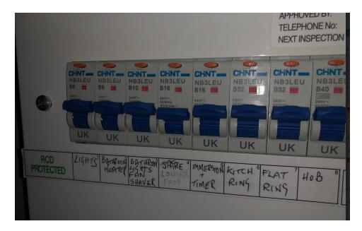
They seldom 'blow' for no reason and an appliance must have caused it. Try and work out which appliance is causing the issue, using the labels and then stop using it. If this does not resolve the issue please contact your landlord.
