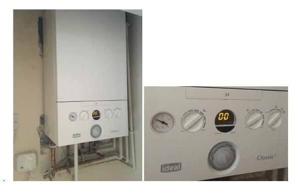
The heating can be set to come on by adjusting the timer (large grey central dial) on the front of the boiler. Use the right hand dial to switch the boiler on and off and for heating/hot water or both. The thermostat for the property is found in the hallway, to the left of the bedroom doorway.
