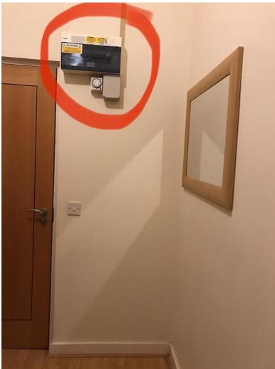
These circuit breakers are designed to cut out rather than ‘blow’ like old fashioned fuses did. Should they cut out then push the relevant breaker back up into the ‘on’ position. The fuse box should then look like this....
